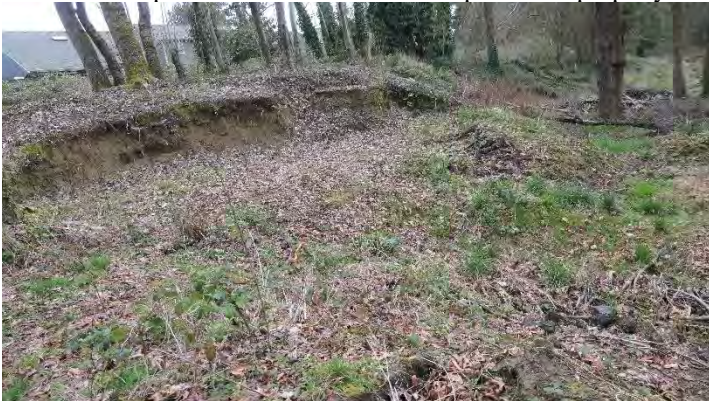
Photo 47. Cut slopes in wetland buffer
