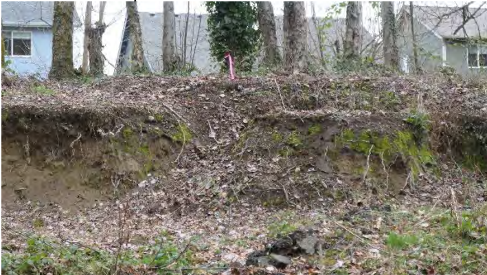
Photo 45. Slopes cut in buffer on northern portion of property
