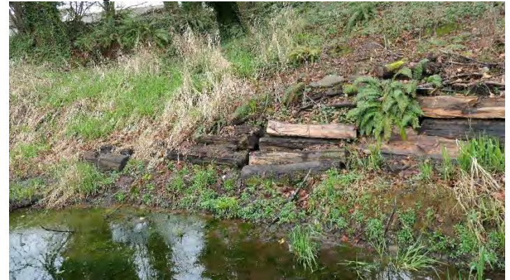
Photo 64. Logs from cut trees used to armor excavated ditch
