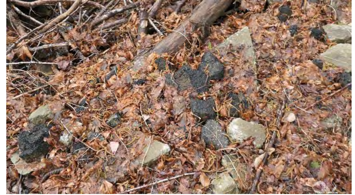
Photo 28. Asphalt, concrete, logs, and fill in wetland A
