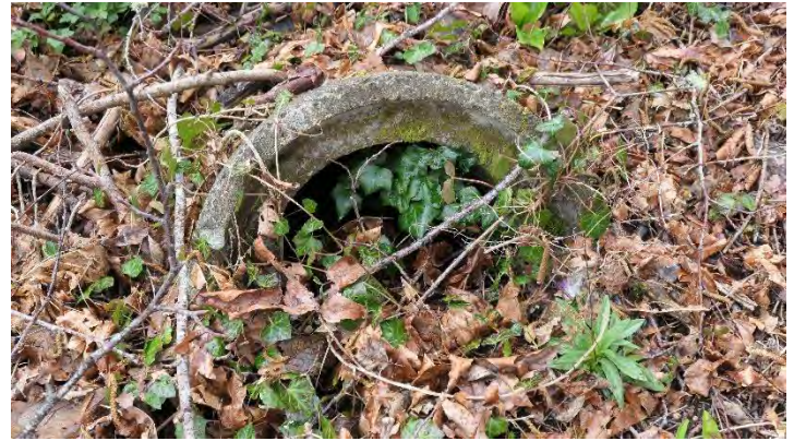
Photo 42. Concrete trash in Wetland A and buffer
