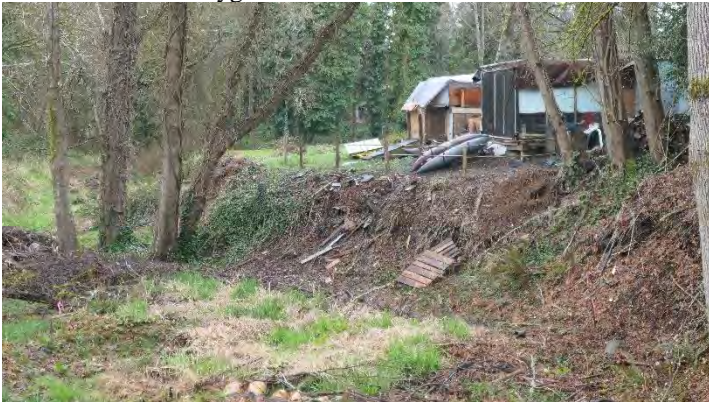
Photo 5. Neighbors appear to encroach onto subject property
