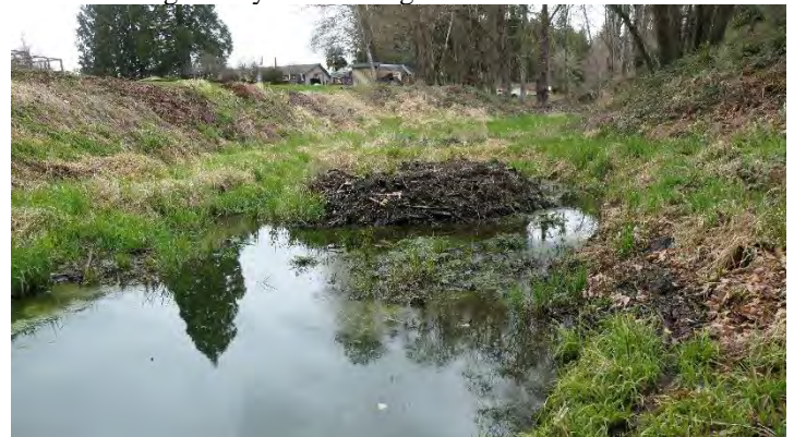
Photo 56. Excavation in southern portion of Wetland A
