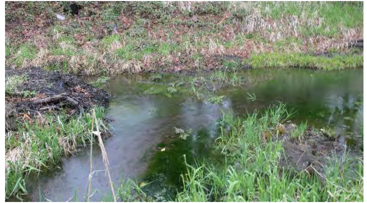
Photo 18. Excavated southern portion of Wetland A
