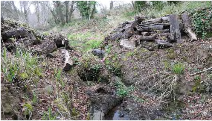
Photo 61. Logs from cut trees used to armor excavated ditch
