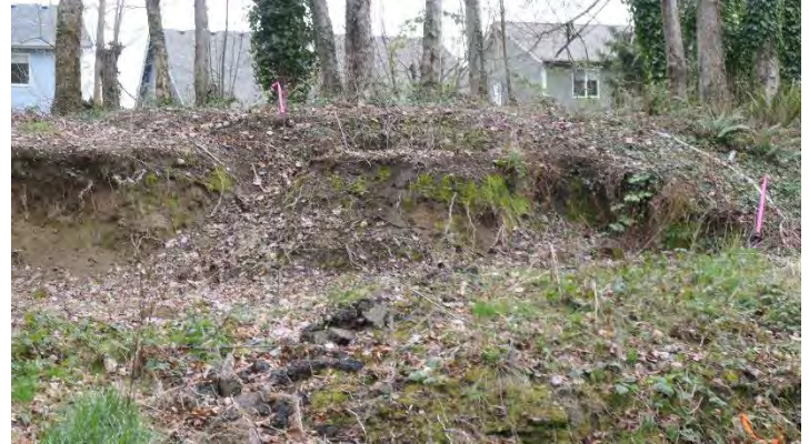
Photo 44. Slopes cut in buffer on northern portion of property
