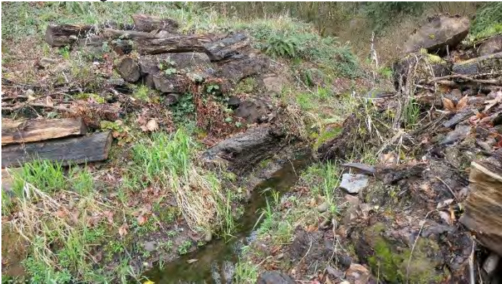
Photo 63. Logs from cut trees used to armor excavated ditch
