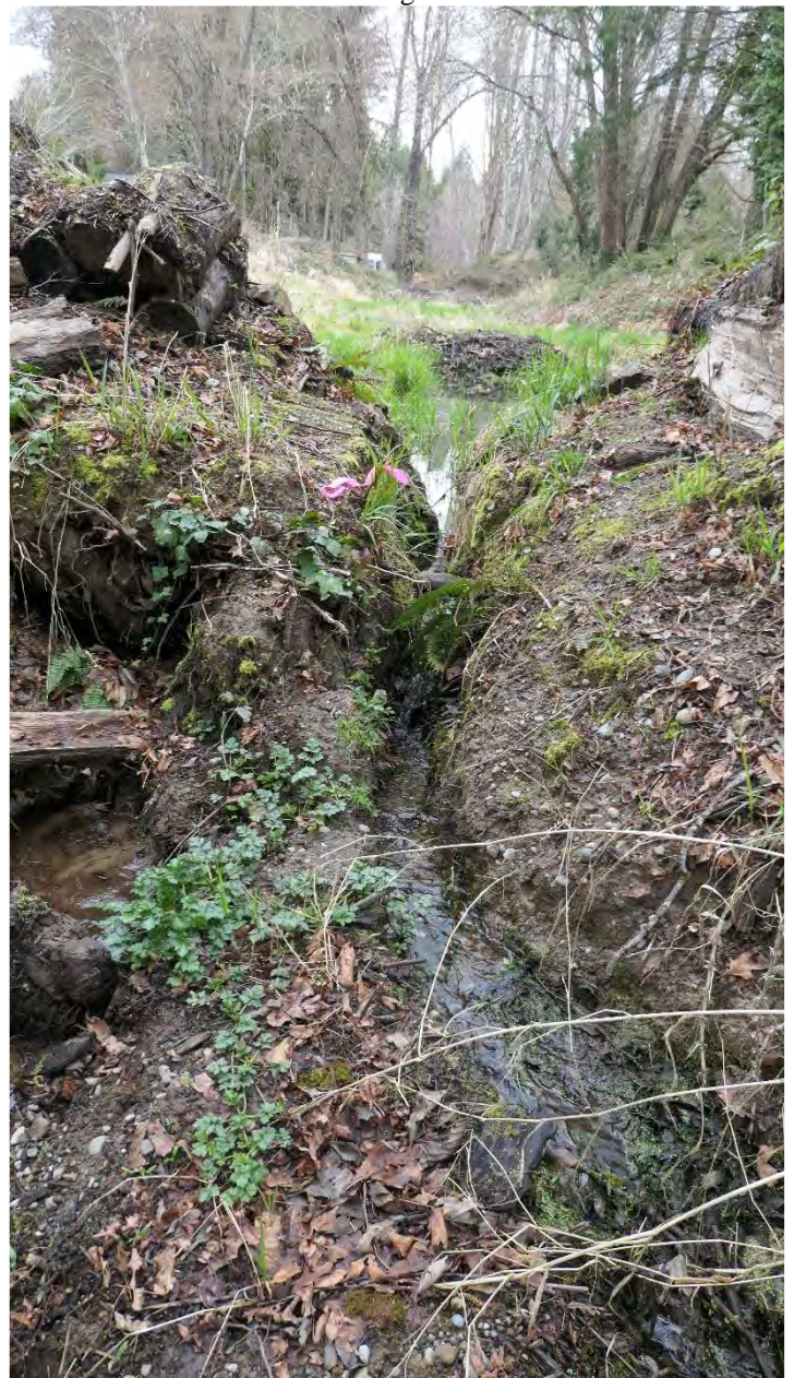
Photo 60. Excavated ditch draining Wetland A
