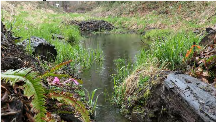
Photo 65. Excavations in wetland to enhance draining of wetland
