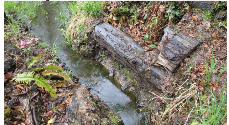
Photo 66. Cut channel and armored bank
