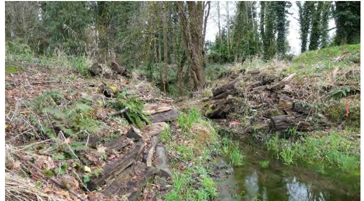
Photo 58. Excavated ditch draining Wetland A
