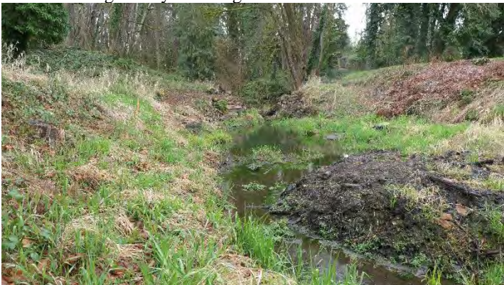
Photo 55. Soils were excavated and placed in soils pile
