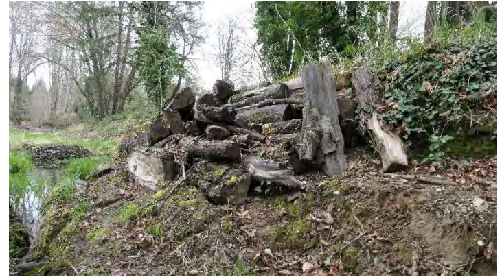
Photo 62. Logs from cut trees used to armor excavated ditch
