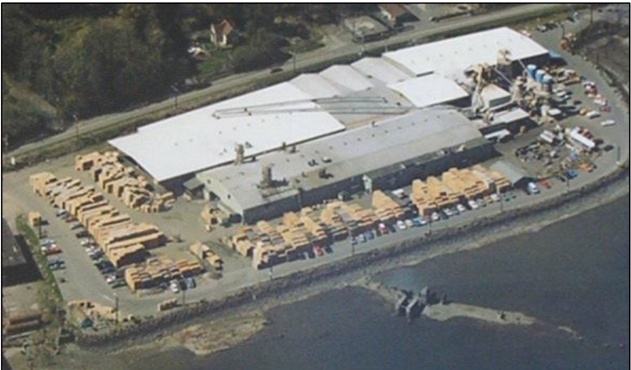
Figure 79. Ca. 1990 aerial detailing the Northern Pacific Tumwater Branch Spurs (TSN: TH2022-1103), view northwest (Moffat & Nichol 2022).
