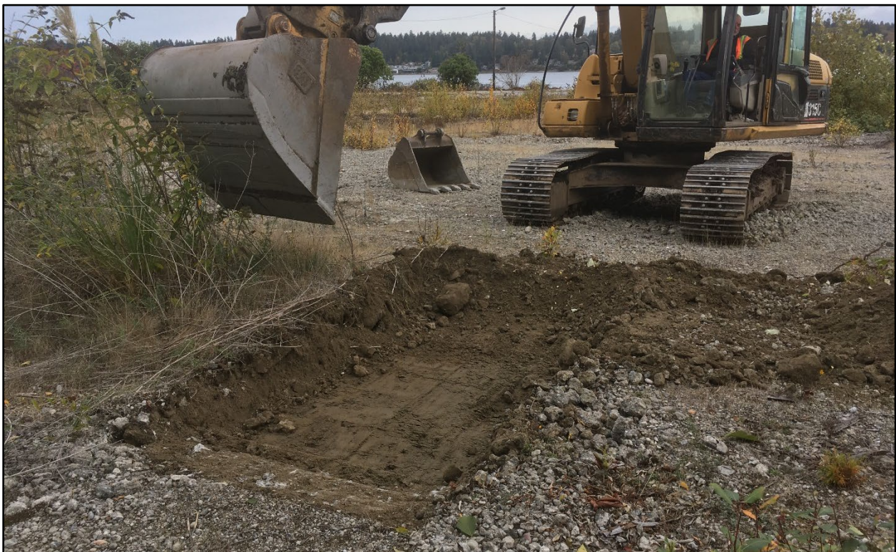
Figure 24. Overview of trench excavation, view northeast.
