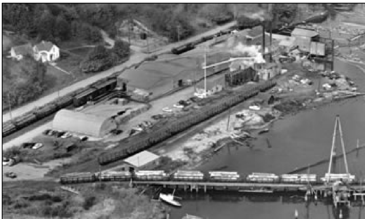
Figure 73. Ca. 1950 aerial of Hardel Plywood Company with railroad cars hauling lumber on the pier, view northwest. Note the three spur lines on the property. Only the east and west lines were identified.
