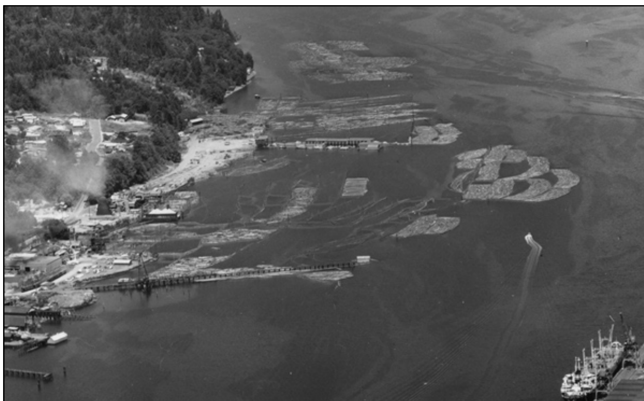
Figure 75. 1967 aerial detailing the Northern Pacific Tumwater Branch Spurs (TSN: TH2022-1103), view is north (Washington State Archives 2023b [cropped by ATCRC]).
