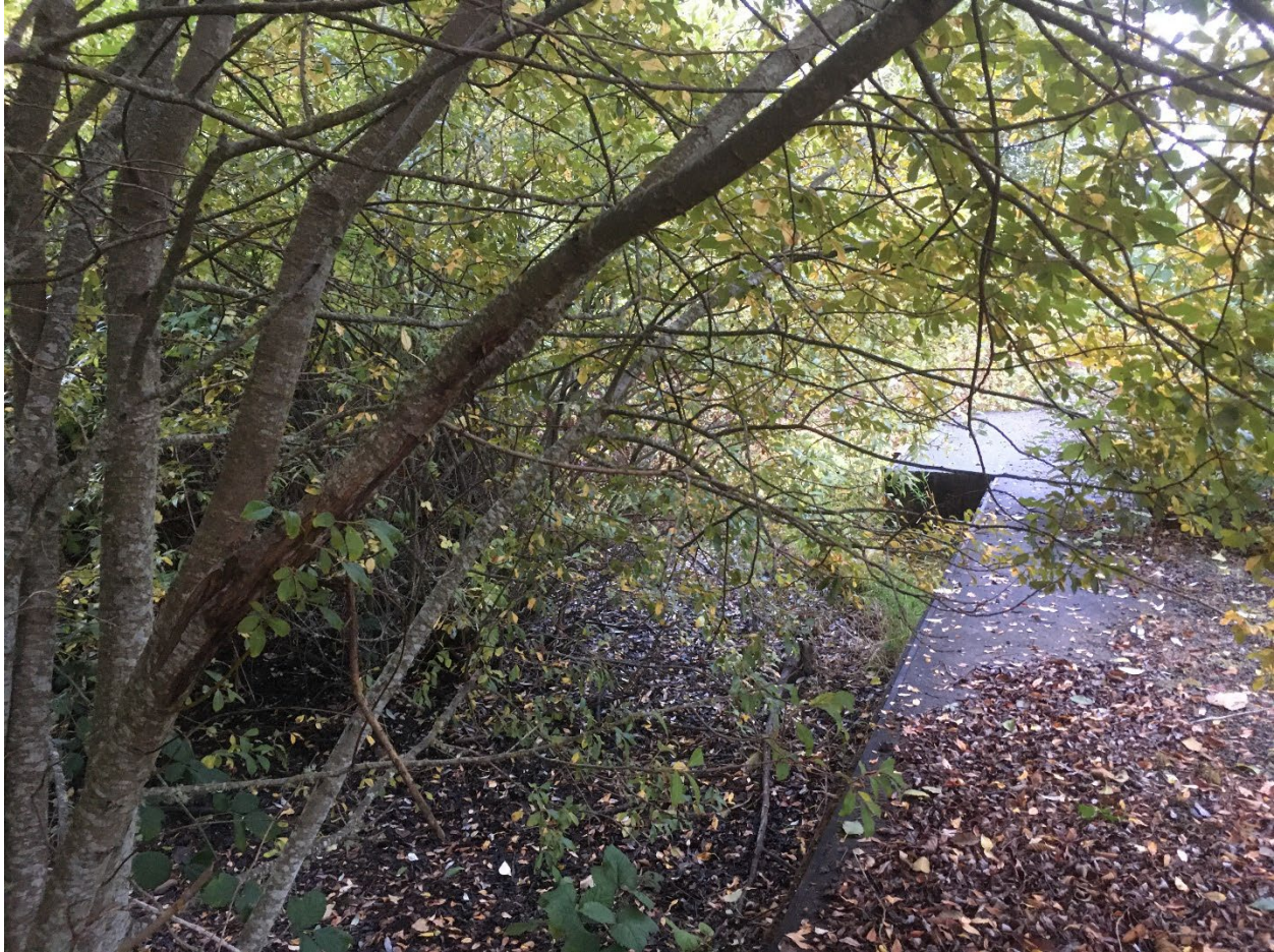
Figure 68. Cement platform adjacent to railroad line in southwestern corner of API.
