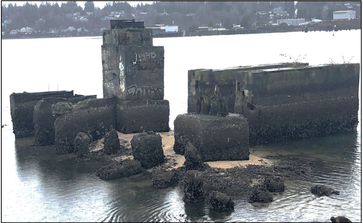
Figure 71. Overview of the piers and concrete platforms for traveling crane associated with the Northern Pacific Tumwater Branch Spurs (TSN: TH2022-1103), direction southeast.
